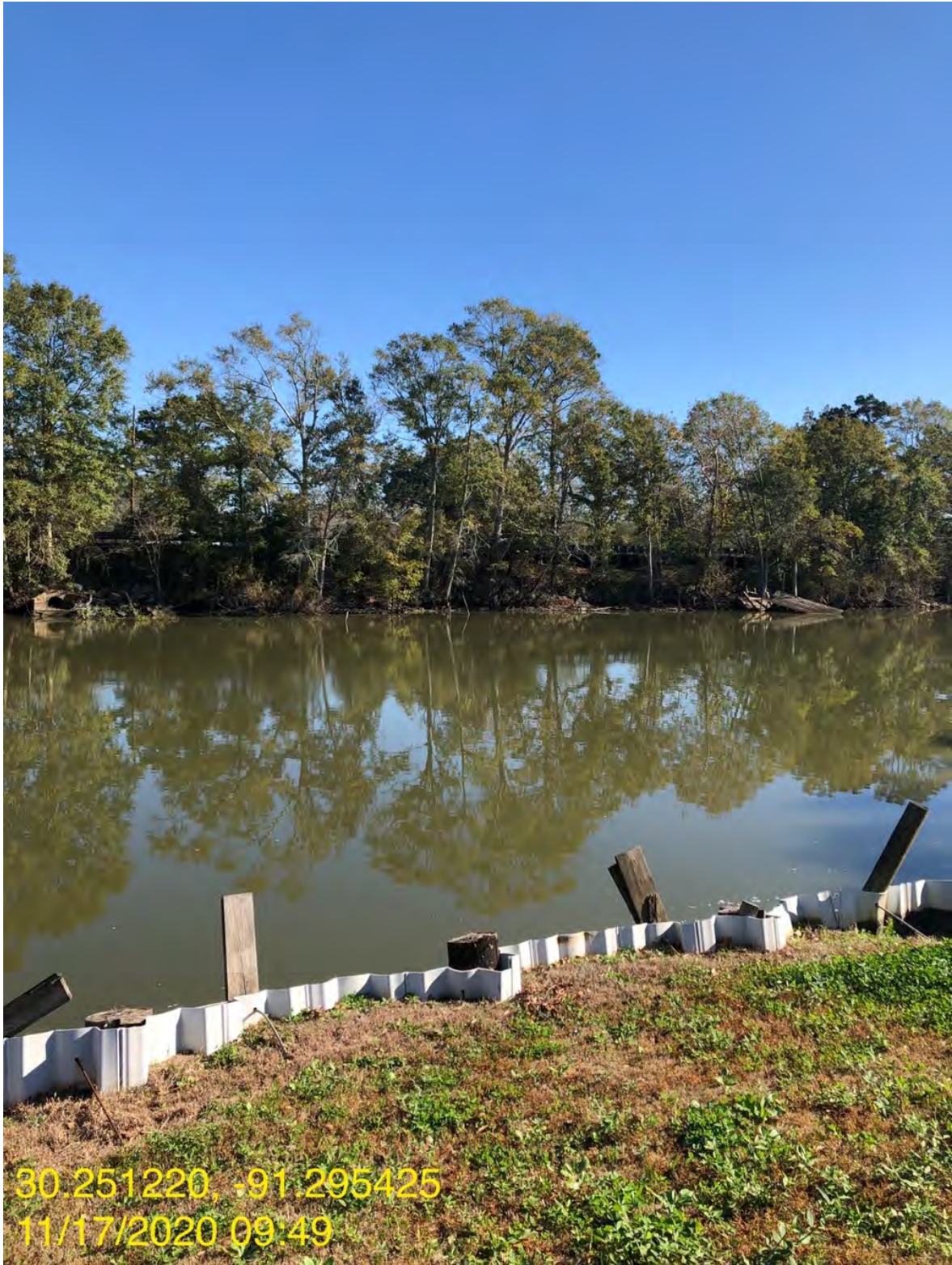
Photograph 6. Facing northeast. Photograph taken on the southern portion of Bayou Plaquemine (Left descending bank) located on the most western portion of the ROW.
