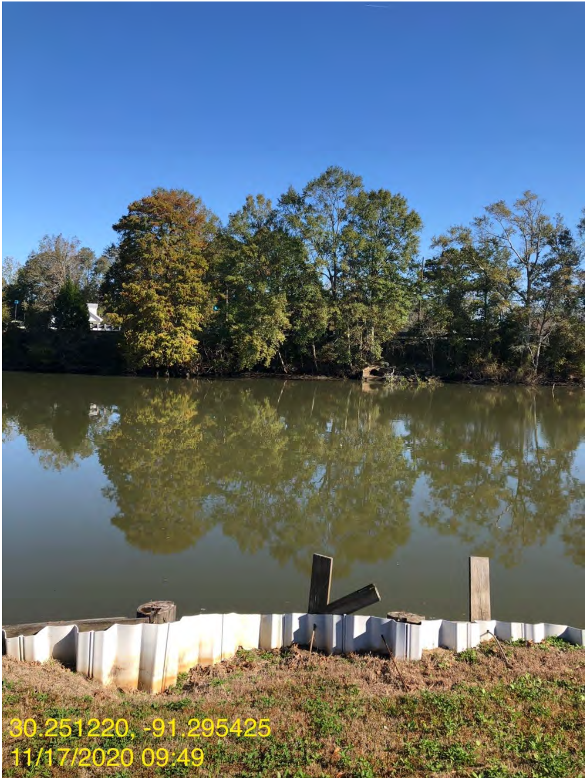
Photograph 7. Facing north. Photograph taken on the southern portion of Bayou Plaquemine (Left descending bank) located on the most western portion of the ROW.
