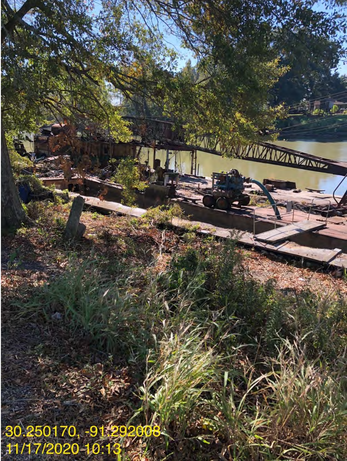
Photograph 18. Facing southeast. Photograph taken on the northern portion of Bayou Plaquemine (right descending bank). Dilapidated barge located within Bayou Plaquemine. A 55-gallon propylene drum and other canisters can be seen on the barge and on land.
