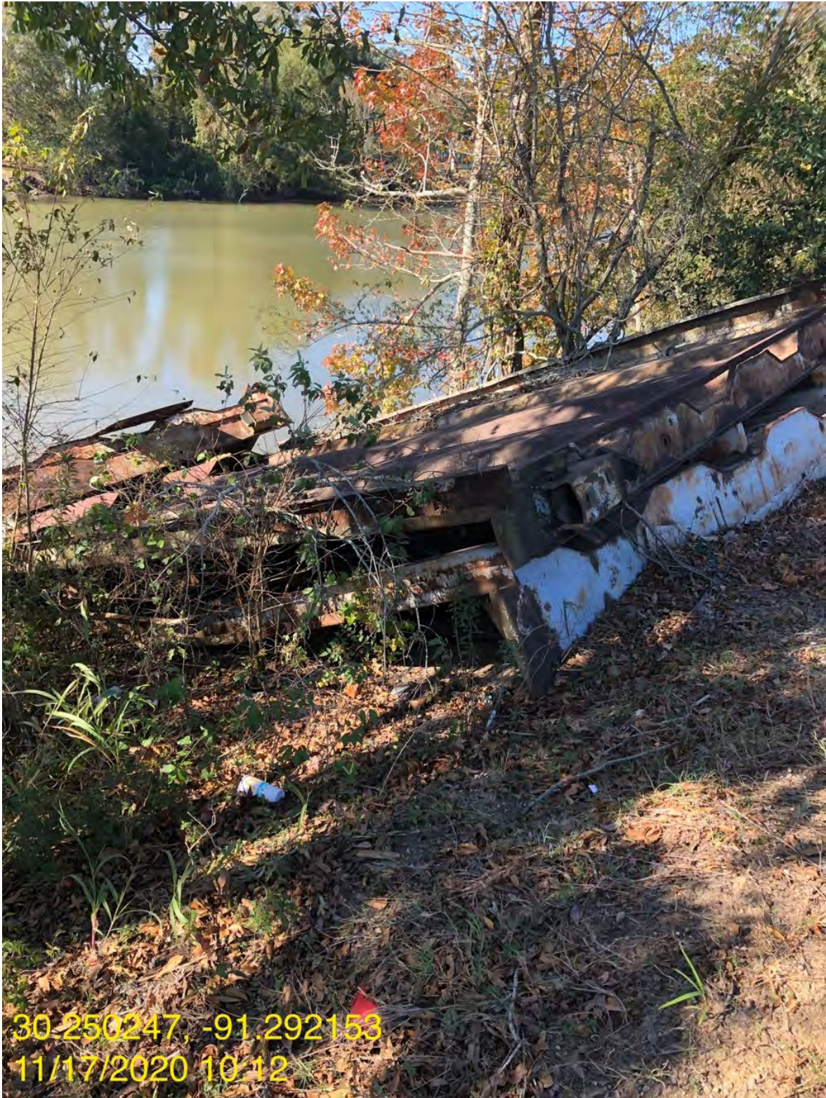
Photograph 13. Facing southwest. Photograph taken on the northern portion of Bayou Plaquemine (right descending bank). Metal support pieces for the dilapidated barge located between Bayou Jacob Road and Bayou Plaquemine.
